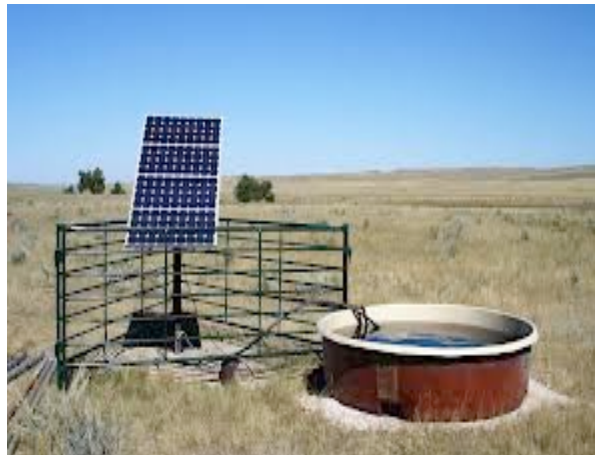
Solar water pumping installation in Namwala
